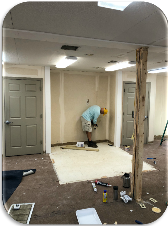
Dirk prepping the walls for paint.
