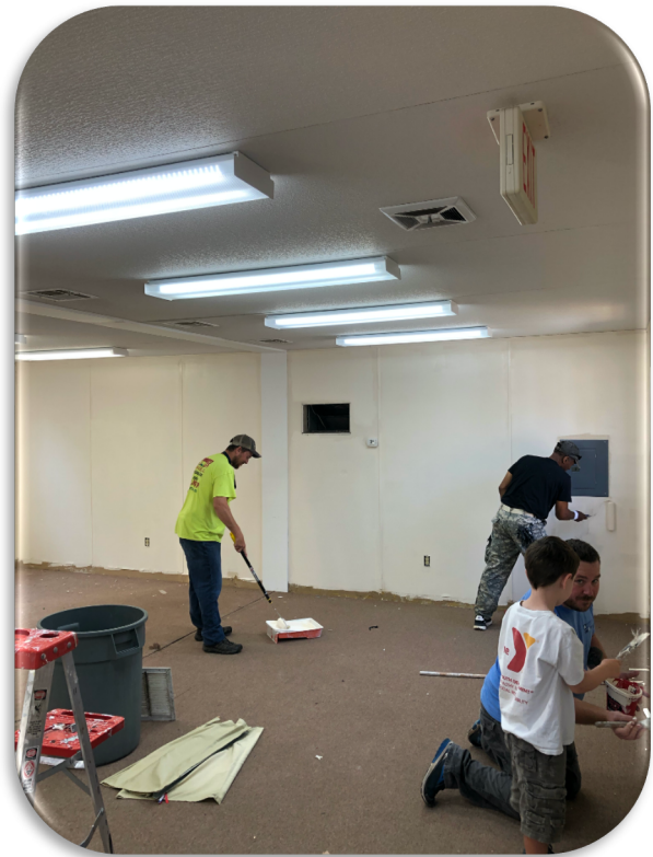
Dustin, Bill, and Joey and Theo getting paint on the walls.
