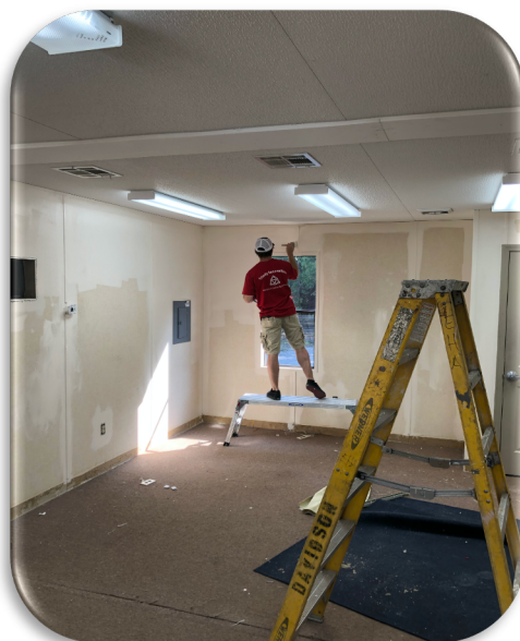
Austin cutting in the second coat.
