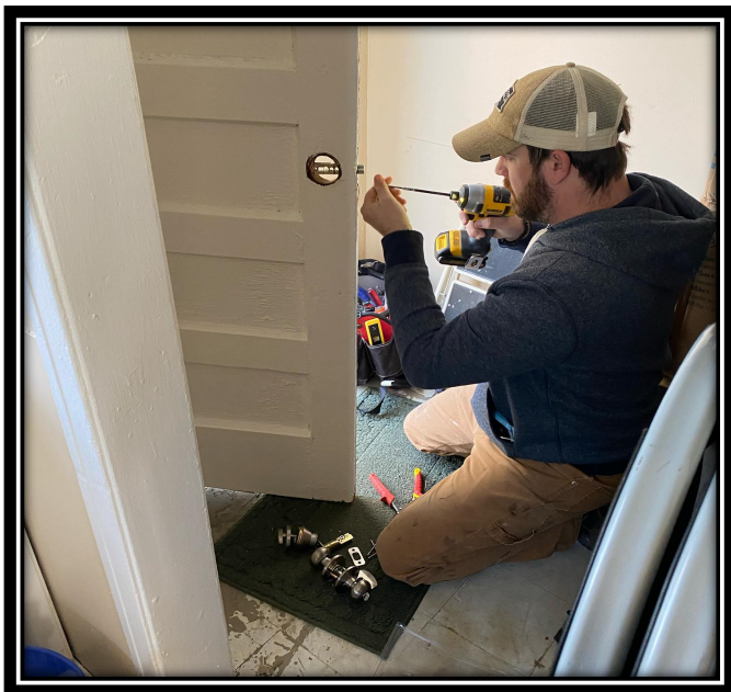
Paul installing new door hardware and locks.
